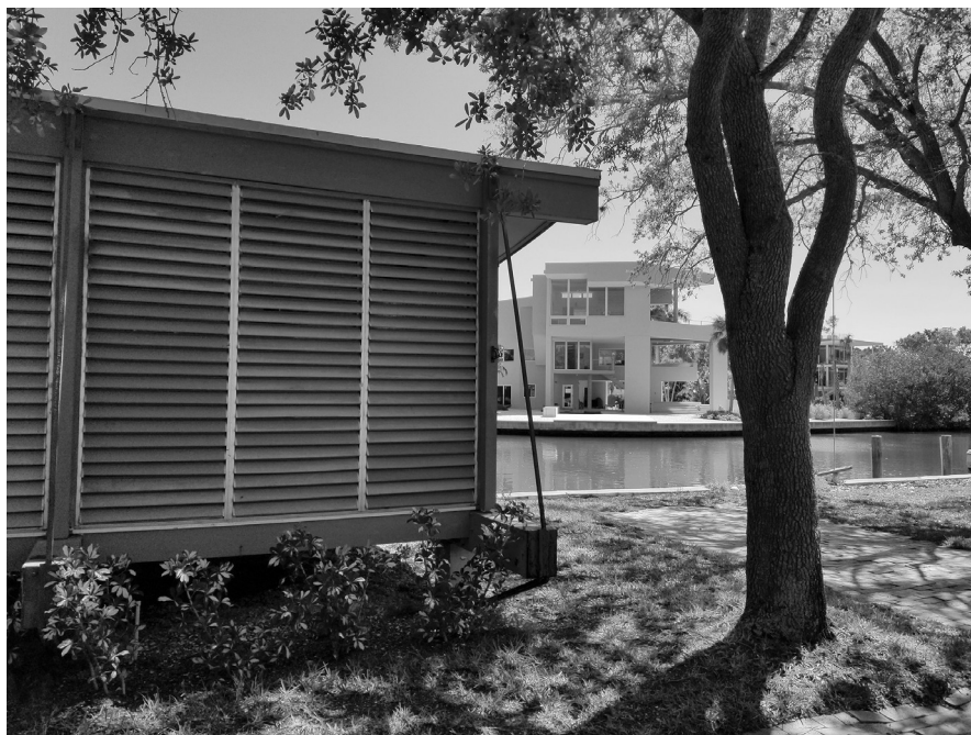
Fig 9. Bayou Louise showing Cocoon House with more recent residential construction in background Sarasota, Florida. Source: Photo by author
